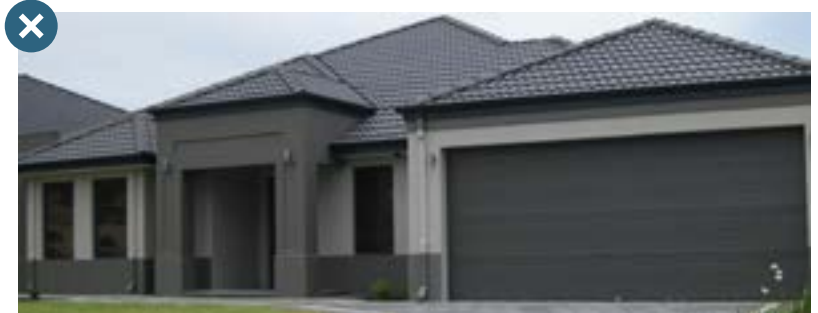
Garage should not be level with house.
